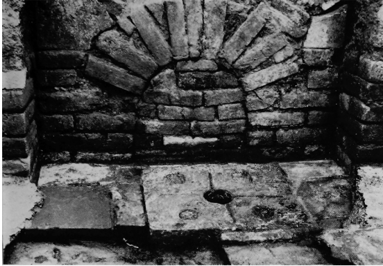
Figure 1 Brick floor, originally waterproofed with bitumen, drain and blocked “man-hole” from the bathing room of the Governor’s Palace, Kalhu (Mallowan 1966, fig. 7)
