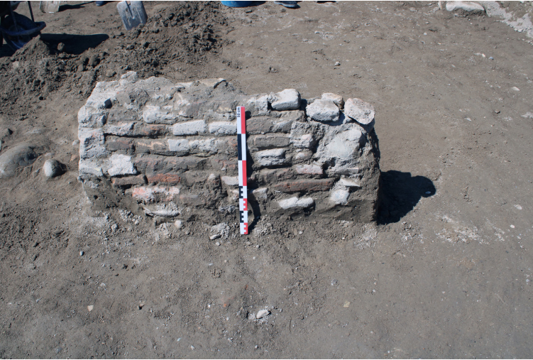
Figure 55 A section of brick wall
