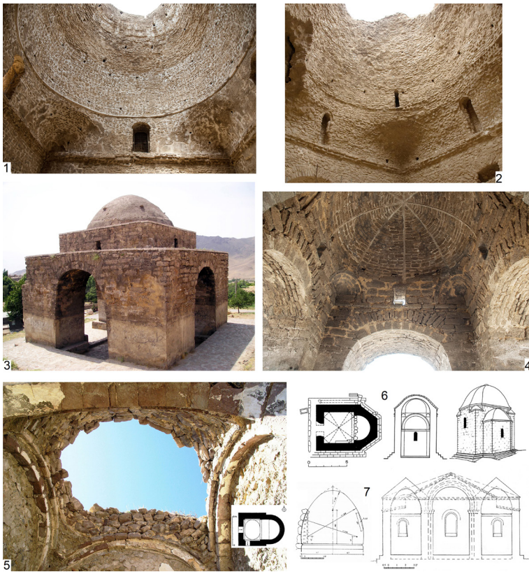
Figure 2 Sassanian and early Christian Armenian domes on square base and squinches.
