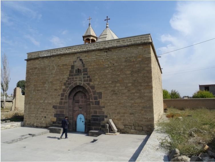
Figure 12 Haftwan S. Gevorg after recent restorations. 2018. © Boriani M.
