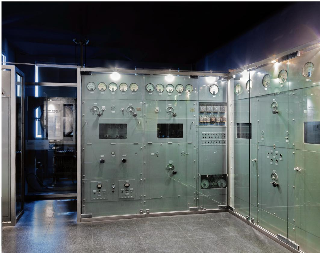
50kW RCA Radio Broadcast Transmitter
