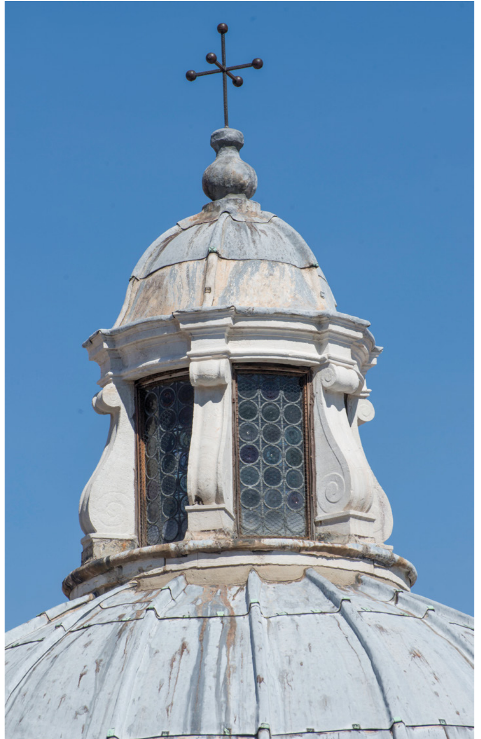
Figure 12 Venice, Rialto, Church of San Giacomo. Detail of the lantern of the dome. Photo © Böhm
