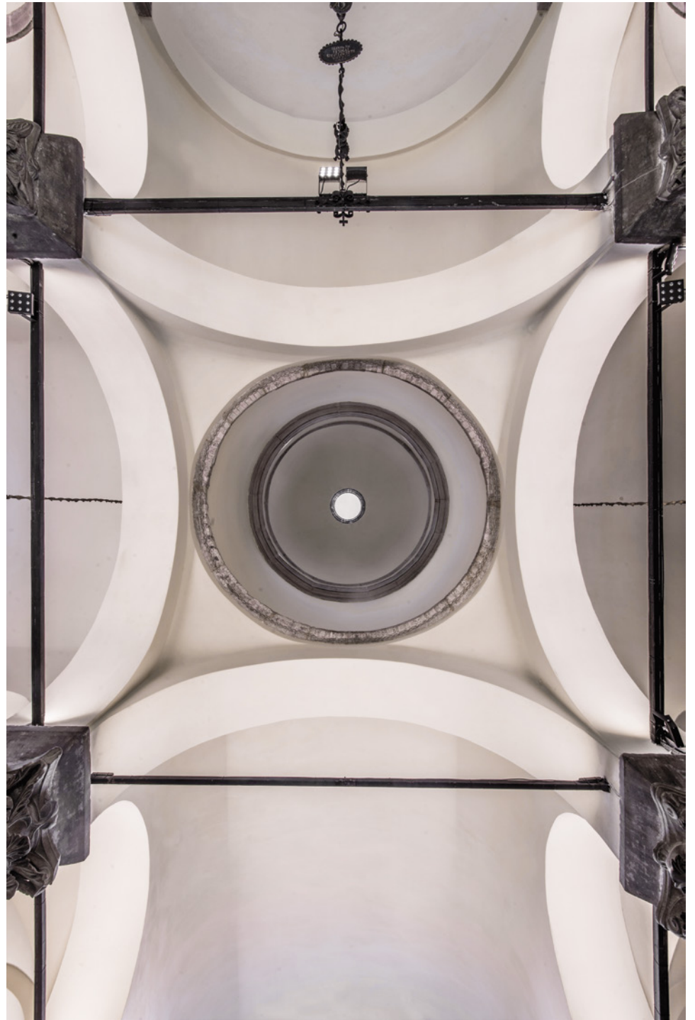
Figure 22 Venice, Rialto, Church of San Giacomo. Inner view of the dome with vaults and arches. Photo © Böhm
