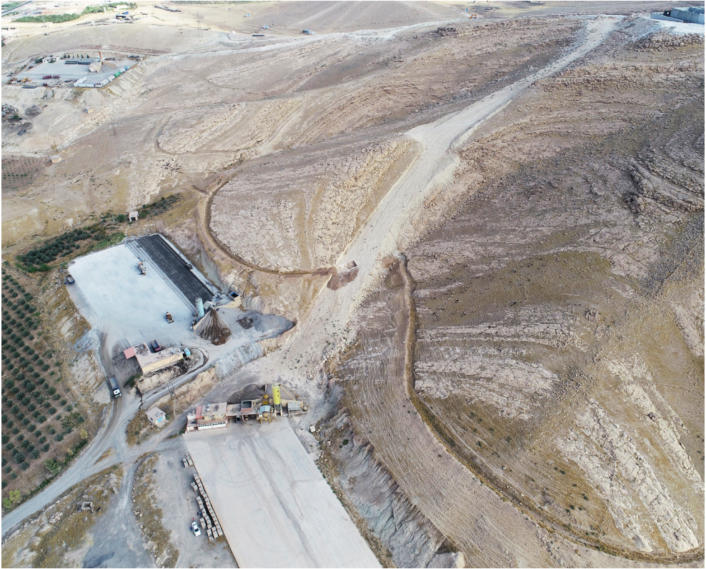
Figure 9 Drone view of three of the four concrete block factories built close to the Assyrian canal at Faida. Note the new aqueduct built in 2018 (top right) and the large trench for housing the water pipe that cuts the canal in two (photography A. Savioli)
