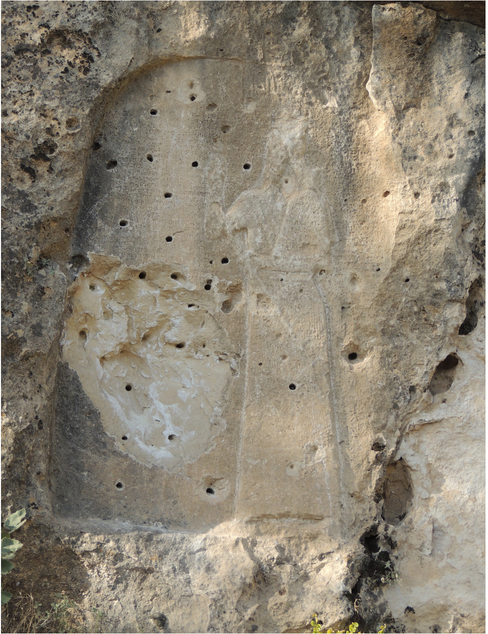
Figure 21b After damage in 2013 (photography R. Orazi)
