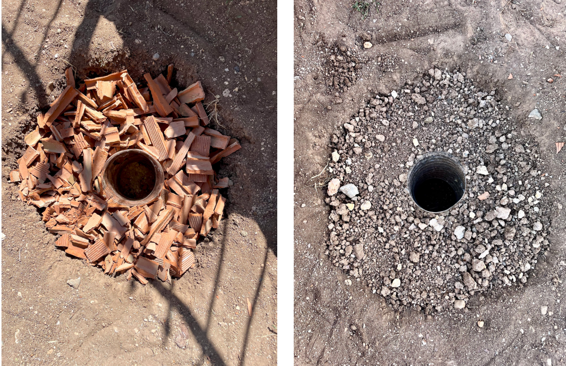
Figure 5 Reconstructed soakaway with brick (left) and soil backfill (right)
